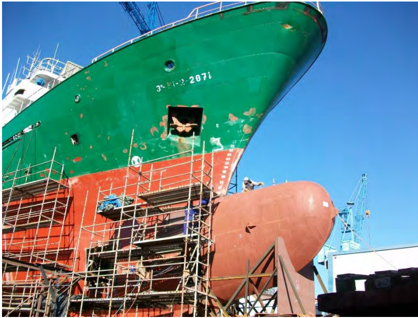
Carbon Steel DH-36 bulb block manufacturing / bending, assembly and welding
